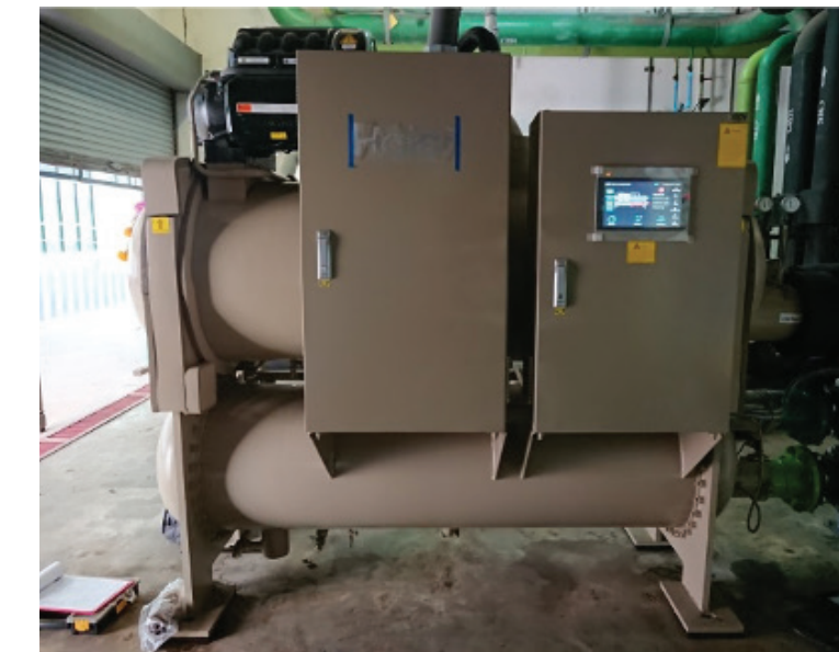
After >> Magnetic Oil Free Chiller Haier kW/ton avg. = 0.505
