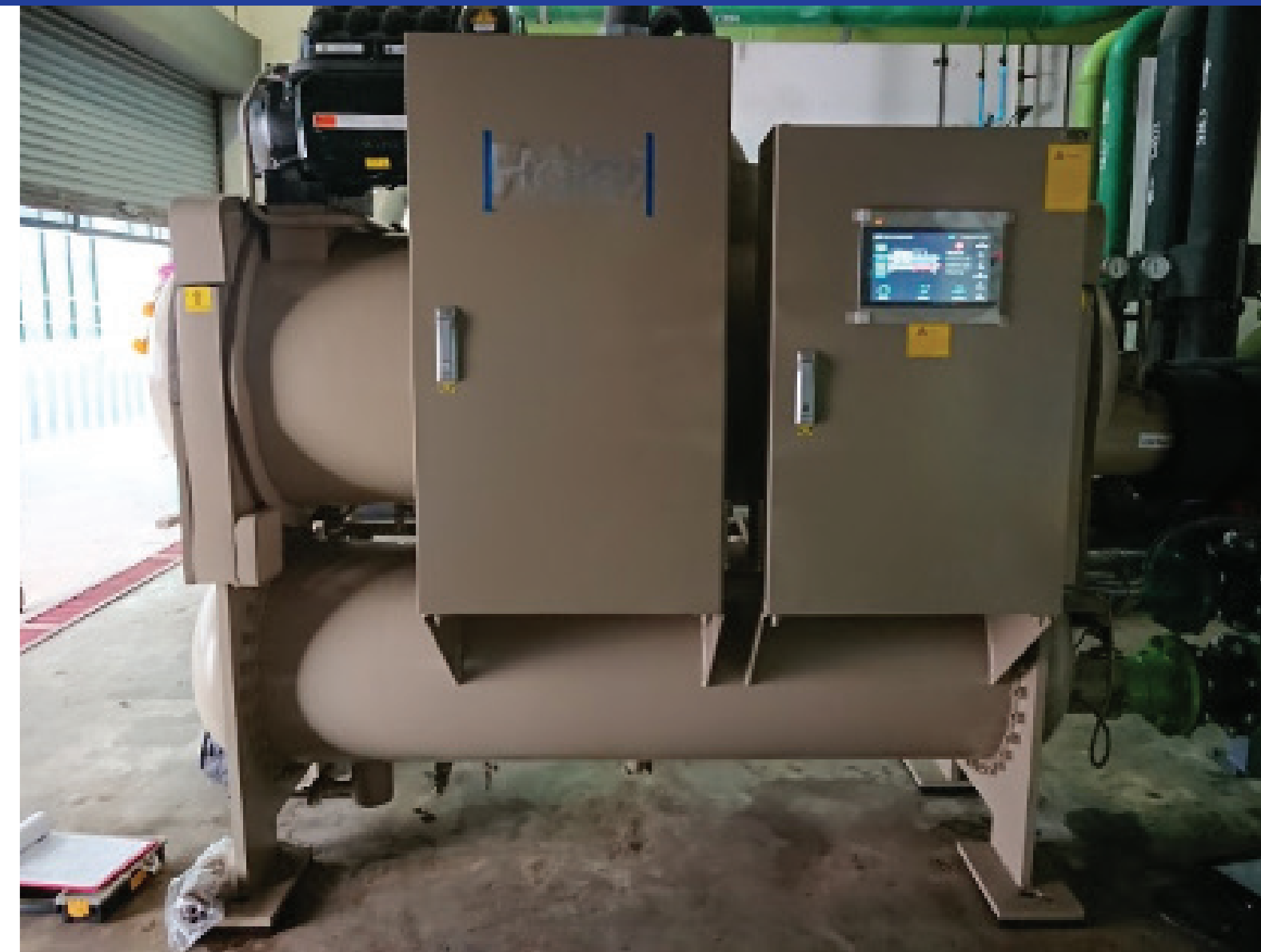
After >> Magnetic Oil Free Chiller Haier kW/ton avg. = 0.505
