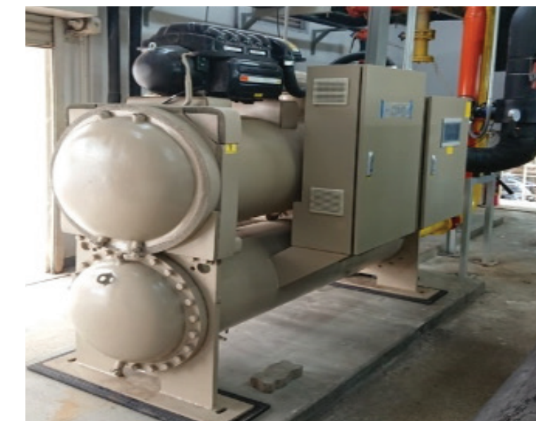
After >> Magnetic Oil Free Chiller Haier kW/ton avg. = -0.554
