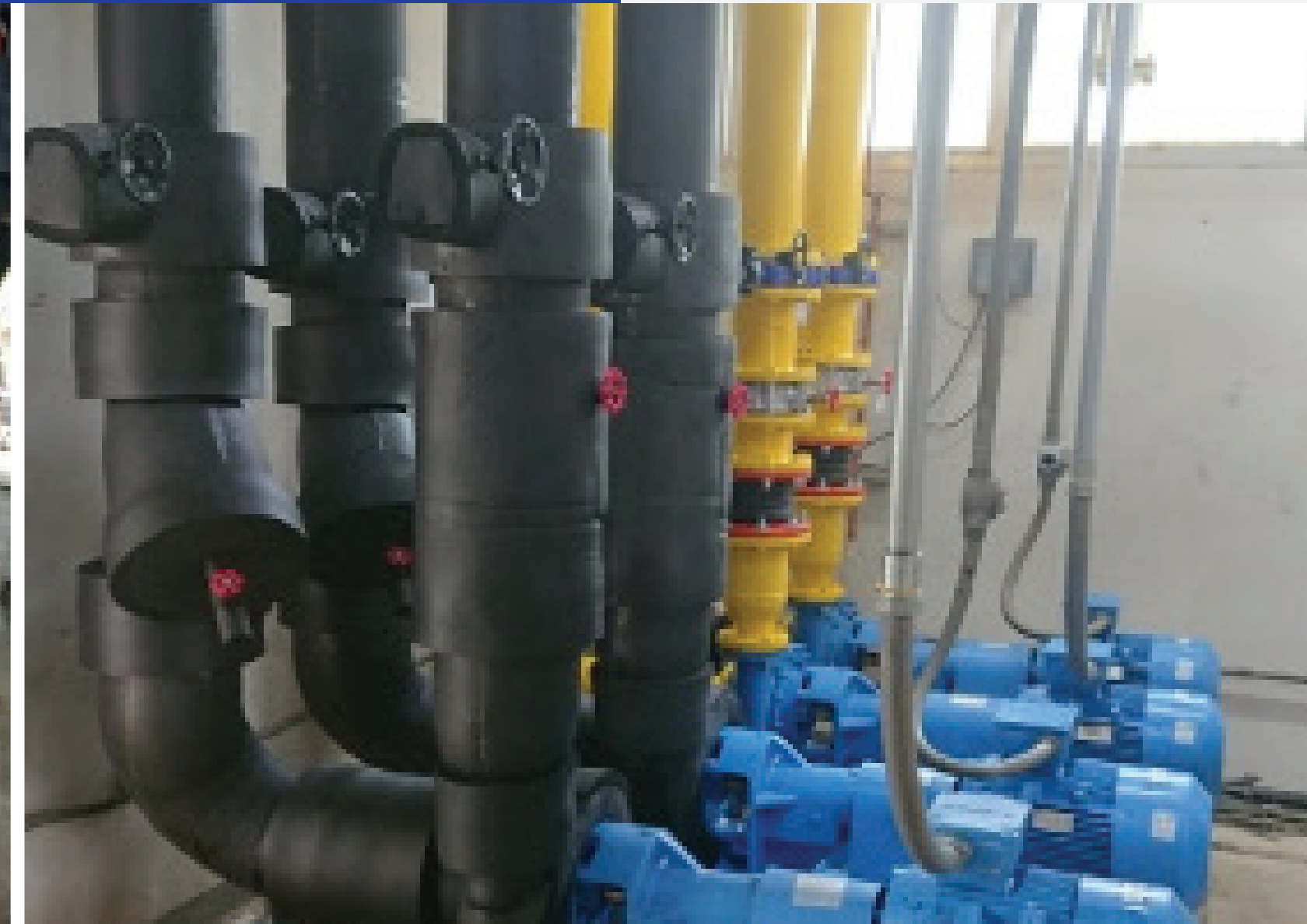
After >> Magnetic Oil Free Chiller Haier kW/ton avg. = -0.554
