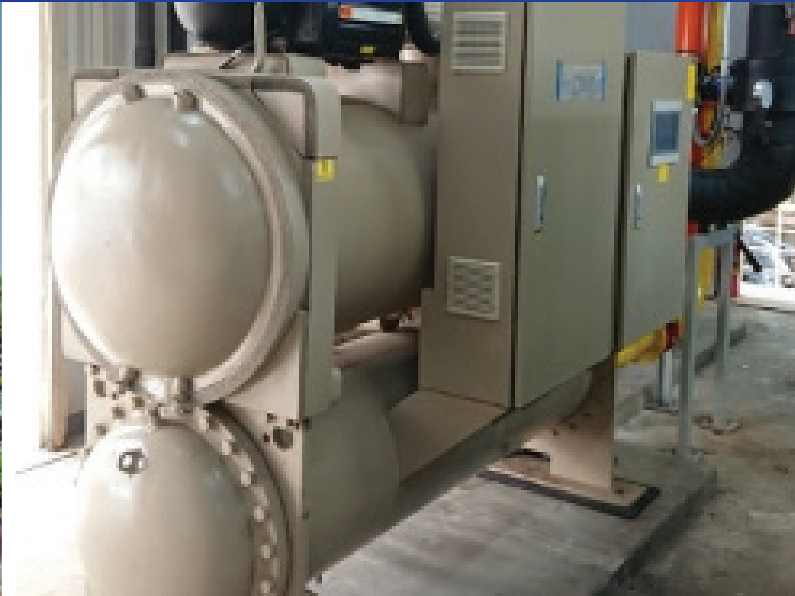
After >> Magnetic Oil Free Chiller Haier kW/ton avg. = -0.554
